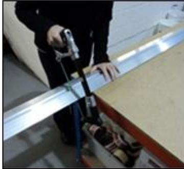
Cut the aluminium section(s) and the two bottom rubber seals to the size of the aperture.
