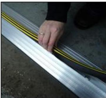
Clean out the channel with a clean cloth to remove excess dirt. Starting from one end of the threshold, pinch the legs of the rubber black and yellow inset and push it in to the top of the threshold until it 'snaps into place'. Continue this process with the remainder of the threshold, taking care to ensure that it is firmly pushed down.
