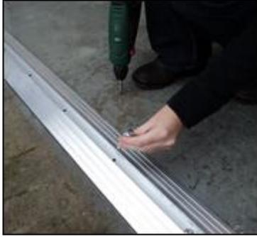
Re-position the Threshold Seal so that the pre-drilled holes in the aluminium seal coincide with the holes drilled in the concrete floor. Starting from one end, place each fixing screw into a hole. There is no need to use plugs as the fixings have a cut thread design that enables them to be drilled into concrete.
