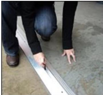
**(Position A)** Position the Threshold Seal in line with the centre of the door so the door will close on the black and yellow cap that runs along the centre of the aluminium section(s).
