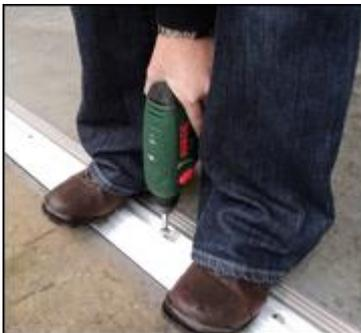
Apply pressure on the Threshold Seal by standing on it. This will compress the two side seals. Then tighten the fixing fully.
