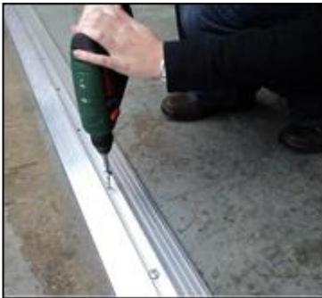
Using an electric screwdriver with the screwdriver bit T30, tighten the fixing until the screw is approximately 5 mm from going all the way in.
