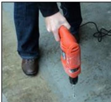
Remove the Threshold Seal and using a 6mm masonry drill bit, drill holes in to the floor where you have marked the ground. (Drill holes are spaced approximately every 200mm and 50mm from each end).
