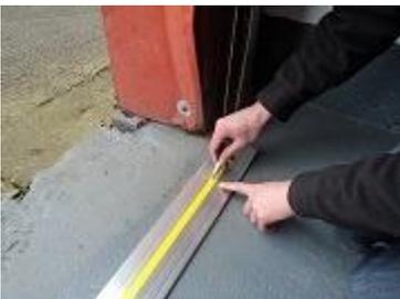
*The holes have been pre drilled in the aluminium for your convenience. The yellow warning tape is designed to cover the holes.*
