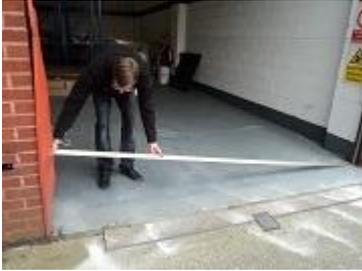
Re-position the Threshold Seal so that the pre-drilled holes in the aluminum seal coincide with the holes drilled in the concrete floor. Starting from one end, place each fixing screw into a hole. There is no need to use plugs as the fixings have a cut thread design that enables them to be drilled into concrete.
