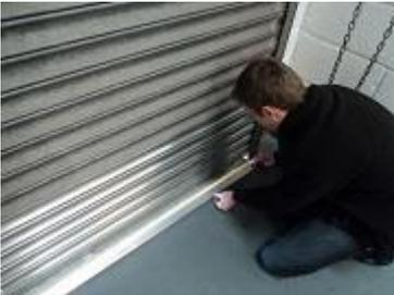
**(Position A)** Position the Threshold Seal in line with the centre of the door so the door will close on the black and yellow cap that runs along the centre of the aluminium section(s).
